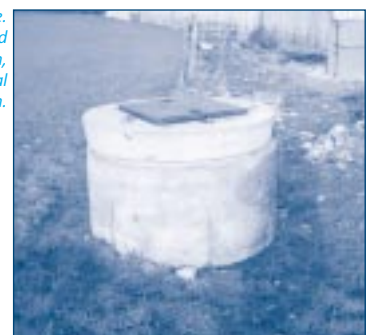
Farm borehole. Good practice above ground headworks completion, upslope of potential sources of pollution.
