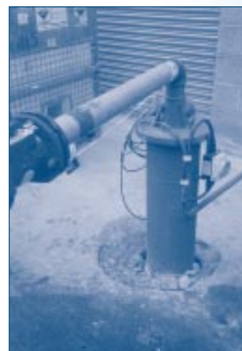
Above ground headworks (good practice) (still to be concreted at ground level), but sited close to stored chemical (bad practice)
