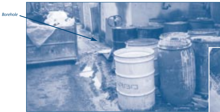
Storage of chemicals and fuels close to and up-slope of a borehole which is completed below ground, with no drain in manhole...
