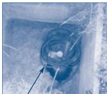
No grout behind casing
